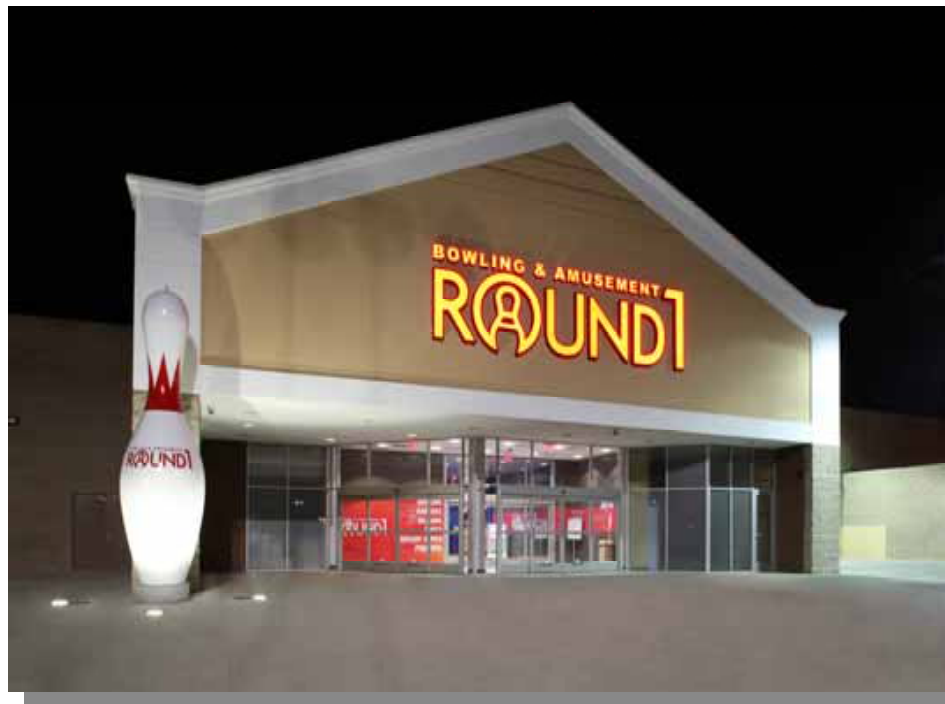
Puente hills mall shop (Los Angeles U.S.A.)
